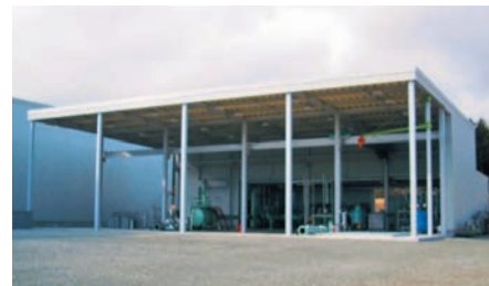
B棟内 開発試験場 Development laboratory in Building B
